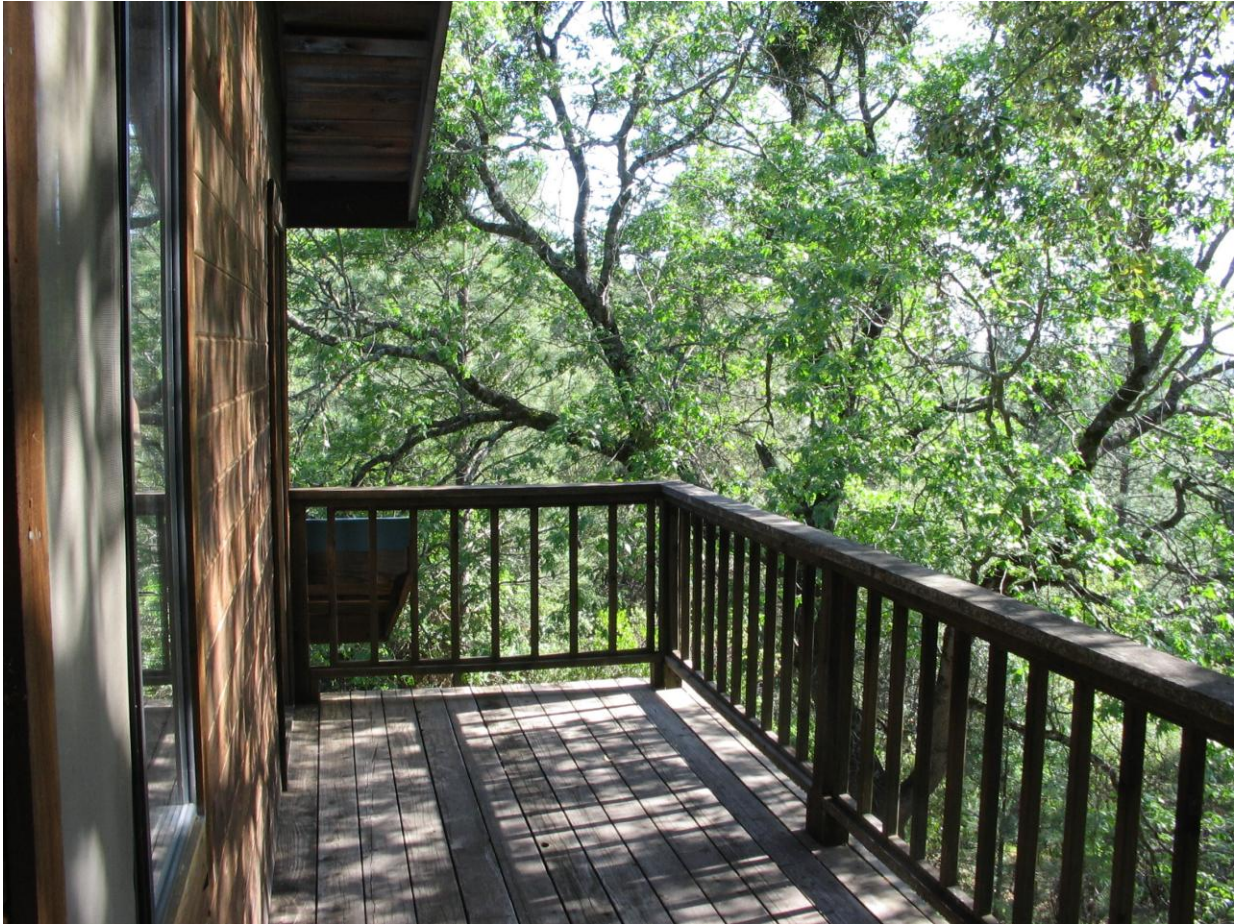
Deck off master bedroom.
